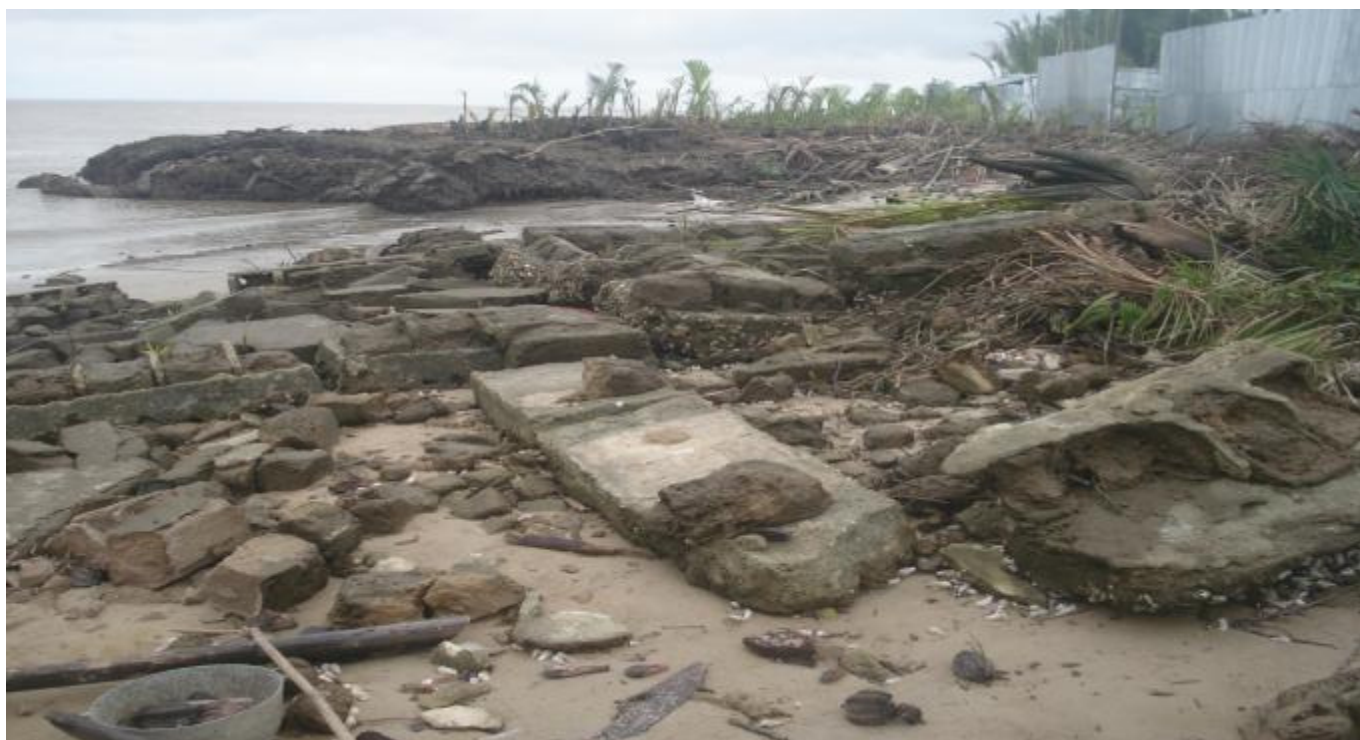
Fig. 1: Debris of Brick Building Destroyed by Sea Level Rise in Ibaka, Mbo LGA, Akwa Ibom State
