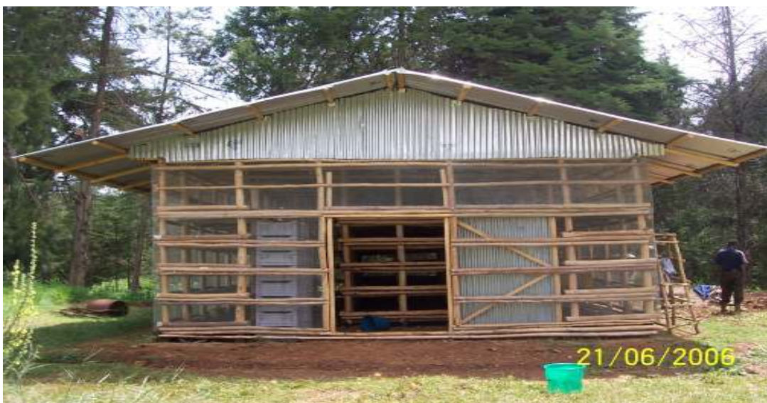
Figure 2 Diffused light store constructed at Holetta research center
