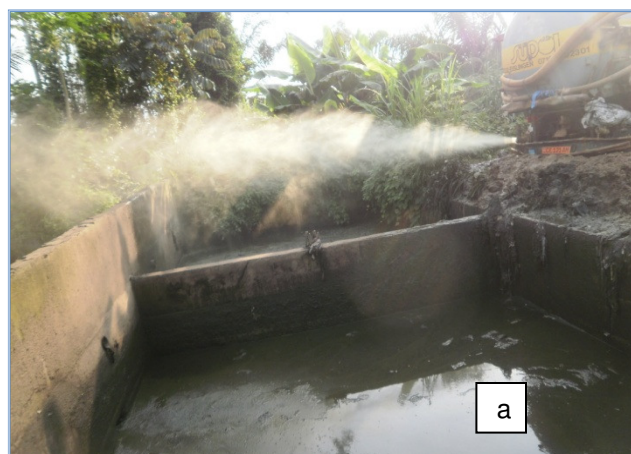
Fig. 1. Partial view of two types of faecal sludge disposal systems at Nomayos, Yaounde. (a) discharge into a well, (b) direct discharge on the ground.
