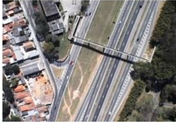
Figure 6 - Original Image Captured by the UAV.
